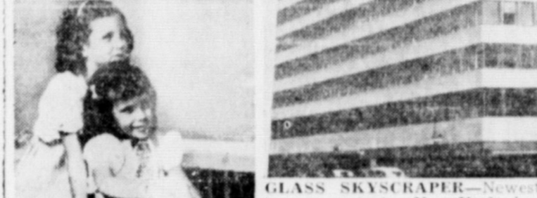
GLASS SKYSCRAPER —Newest tower puncturing New York skyline is shimmering Universal Pictures Bldg., whose 30,000 square feet of glass, according to Libbey-Owens-Ford, projects daylight a record 40 feet into its interior.
