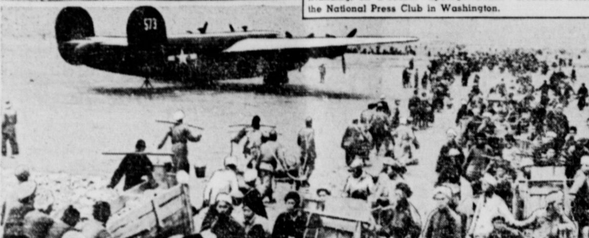
MANPOWER! —With shortage of modern gear, this battalion of Chinese laborers uses time-honored methods in carrying rockpile (lower left) to airfield to be used as runway bed for our fliers fighting the Japs from Chinese bases.
