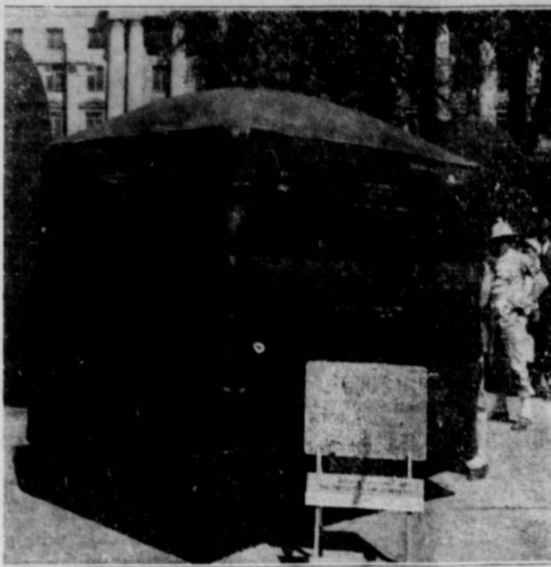
Typical of the wartime tasks assigned to cotton is this newly developed "pneumatic lift," used to hoist planes landed in rough terrain. Made of rubber-coated cotton fabric, the bag expands to the size of an average small room or office when inflated. Used in pairs, the bags can lift the largest Fortress bombers off the ground.
