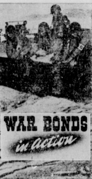
On the beaches of Italy, in the jungles of the Pacific—planes, tanks, artillery must move—and fast; no waiting to build roads or airfields. That's when our soldiers must unroll these "steel mattresses," as you see them in this photo. Your War Bonds pay for them. U. S. Treasury Department
