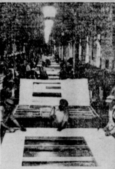
PRECISION HOMES —These workmen at Libbey-Owens-Ford Glass company are placing material on walls for precision built pre-fabricated homes made by the company under government contract to help meet acute housing shortage for industrial war workers.
