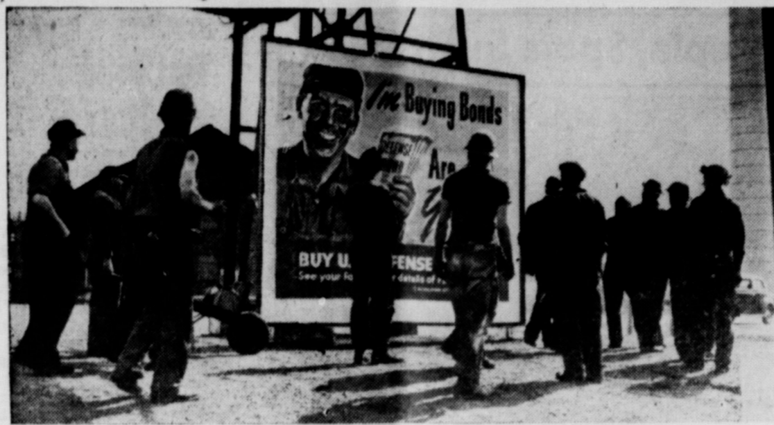
At the Bethlehem Steel Corporation plant, Bethlehem, Pa.
