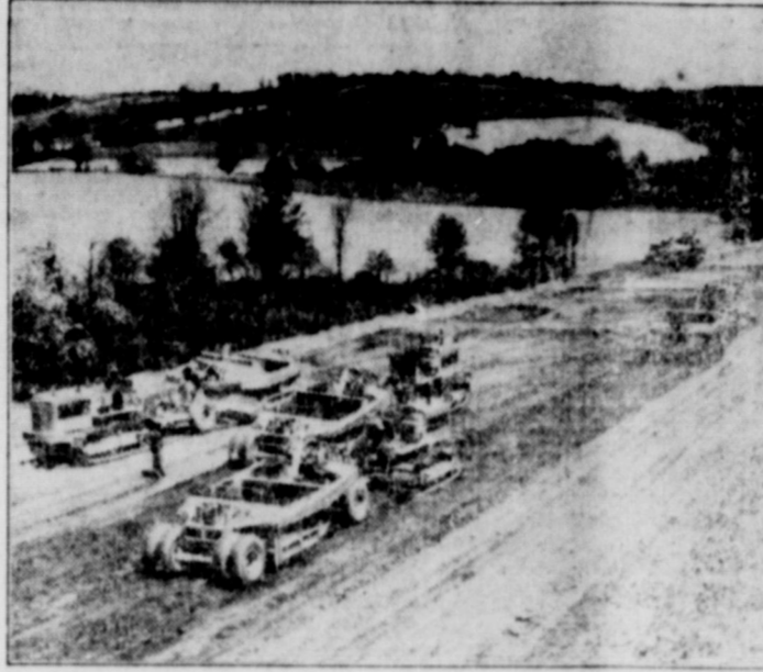
Fleet of huge tractor drawn, hydraulic scrapers hurry to meet July 4th opening date of the Pennsylvania Turnpike.
