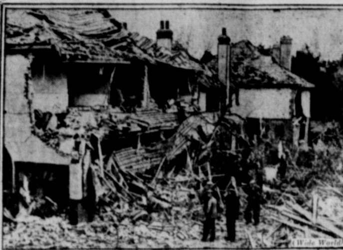
WHEN BOMBERS FALL . . . Whole row of houses at Clacton-On-Sea, England, was wrecked when huge German bombing plane crashed and exploded, killing five persons, four of them crew members, and injuring 90 residents.
