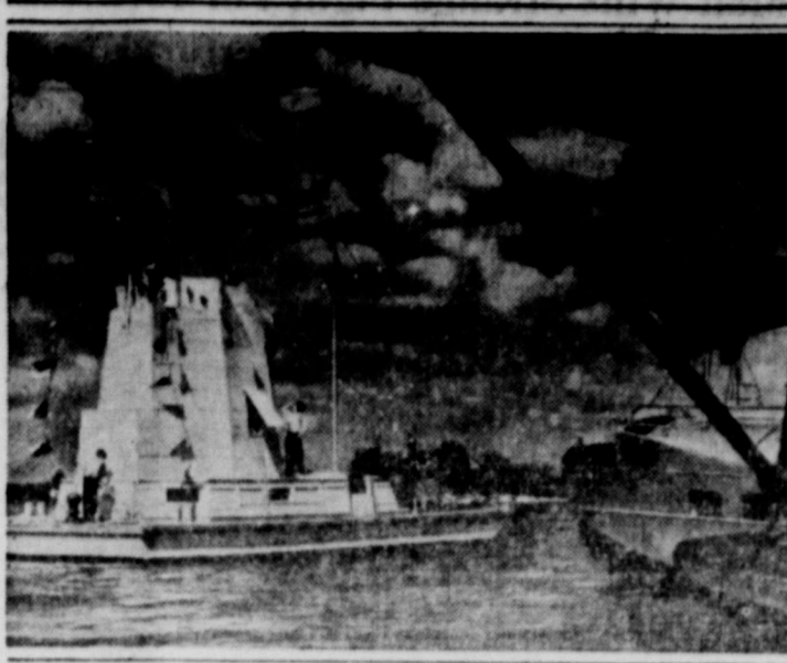
Designed by Mr. J. E. Williamson, noted marine explorer, the Williamson Photosphere, stationed at Nassau, the Bahamas, is equipped with a huge flexible tube which lowers the large photosphere down through the great well of the flat-bottomed craft for observation of undersea life, seen through the five-foot window. A special camera takes motion pictures of the varied types of fish and undersea vegetation. Close by the photosphere is one of the giant Pan American Airways flying clippers which this winter are operating on a daily schedule between Miami and Nassau.
