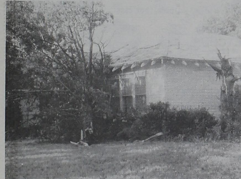
A LARGE CEDAR TREE on the north side of the Mickey Jackson home apparently was lifted up and over the corner of the house, landing on the east side, and jammed under and on top of their front porch. Several wood pieces were left sticking in the roof.
