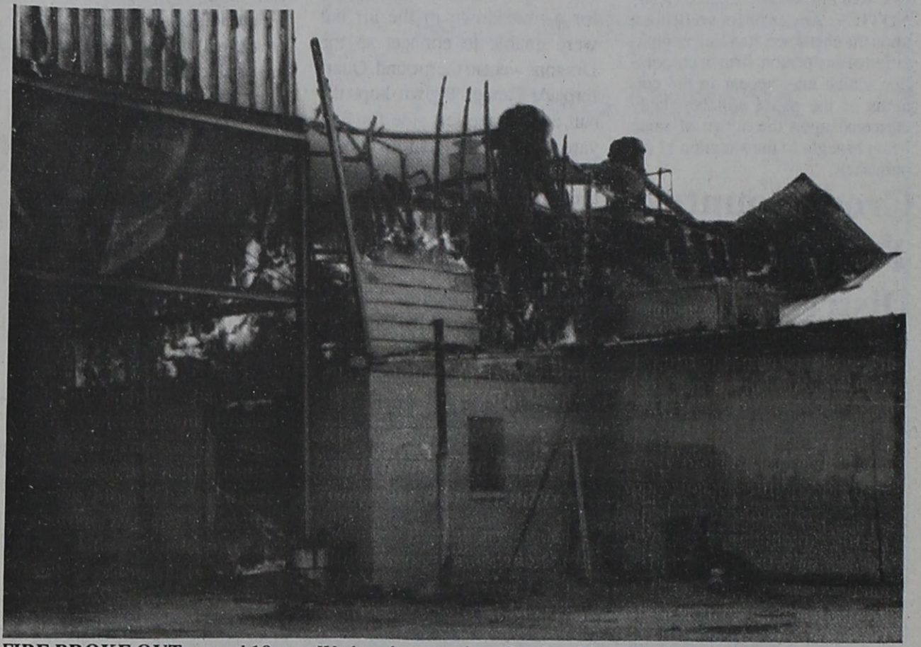
FIRE BROKE OUT around 10 a.m. Wednesday morning, October 14, at Abell Ag Co. Local firemen were quick to arrive at the scene and distinguish the blaze. Clean-up and reconstruction has already started, and the plant should be back in shape for cotton season within thirty days. Electrical wiring trouble is guessed to be the cause of the fire.
