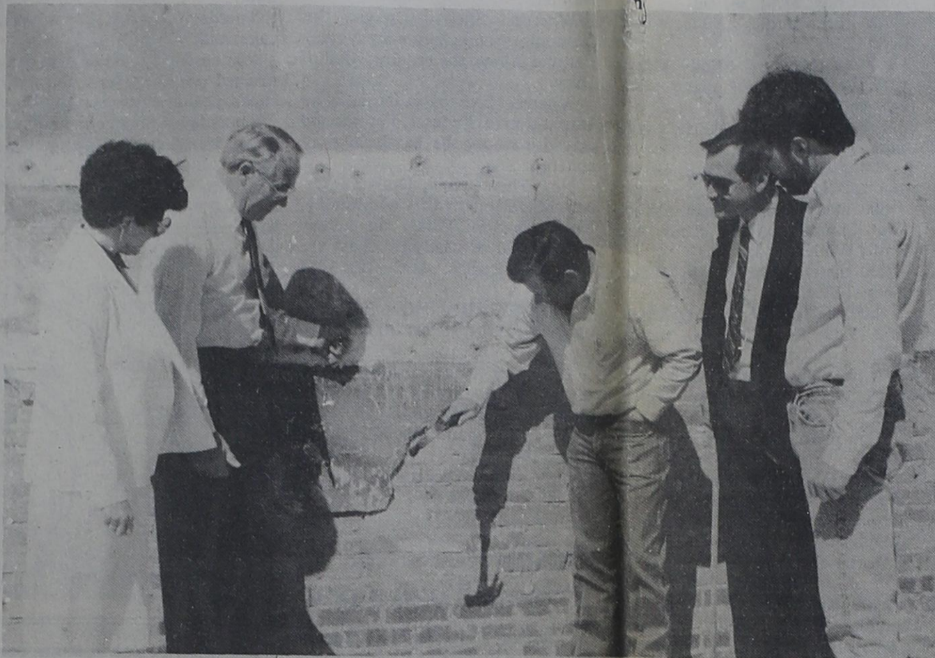
IT'S HARD WORK, BUT... Steve LeFevre, center shows a group of Chamber of Commerce members the easiest way to break plaster off the brick wall in the burned out area in Munday's business district. From left, Ronnie Cude, Charles Baker, Lyndle Reeves and Perry Kuehler will join others for a workday at 5 p.m. Thursday to chip the walls and remove old tile from the floor. Anyone willing to help in this project is asked to bring tools, goggles and plenty of energy to assist in getting this area cleaned up.
