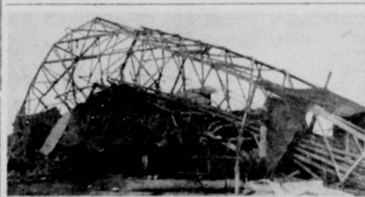
One man was seriously injured and three others had narrow escapes when this drilling rig collapsed on the Underwood lease west of O'Brien early Monday.
