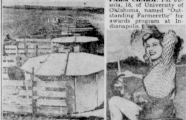
PIGLOMS like these feature new isolated-birth system developed by Nutrena Mills and expected to revolutionize hog-raising methods, greatly reducing piglet loss from disease and crushing.
