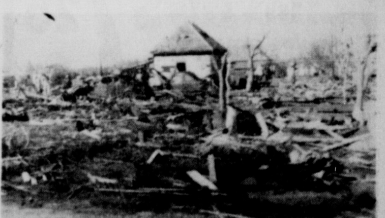
ONLY DEBRIS remains where the northeast part of Knox City, once stood two houses, the in the area where three persons homes of Mexican families in were killed.
