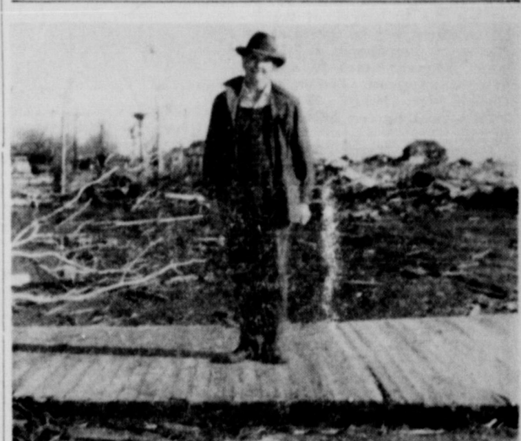
PORCH BUT NO HOUSE — Ed Nance is standing on the porch behind which stood his house until Friday's tornado took it as part of its toll. Neither Mr. Nance nor his wife were at home when the storm struck. It was just east of the home where Mrs. L. L. Houston was seriously injured.
