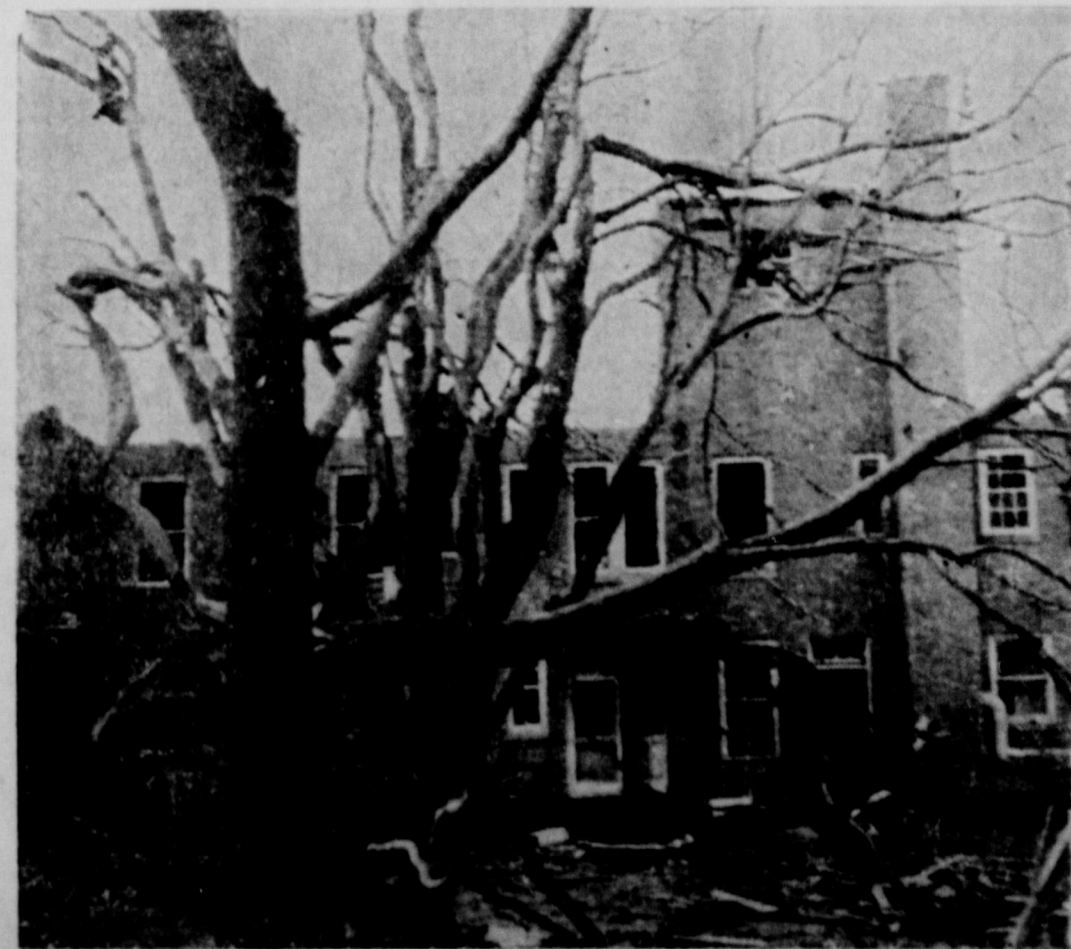
SHATTERED TREES — The battered Knox County Hospital stands behind broken trees and branches, starkly emphasizing the wrath of Friday's tornado. The hospital felt the brunt of the storm but twenty-seven patients and seventeen staff members in the building at the time of the storm were unhurt. Patients were evacuated. (Photo by Bill Baker)
