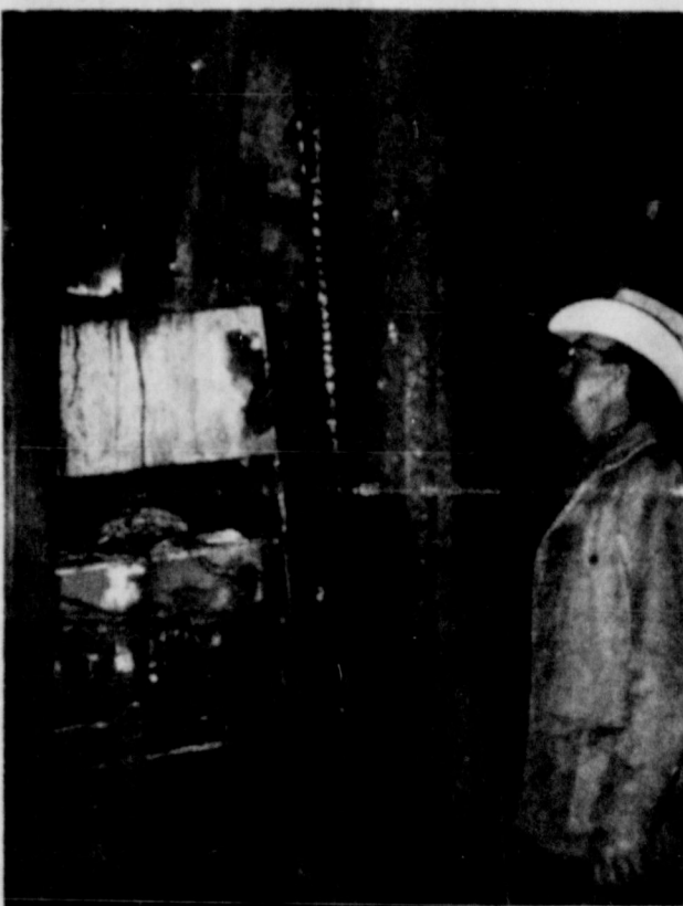
SURVEYING THE EXTENSIVE DAMAGE from last Thursday morning's fire is Knox County Farmers Home Administration's supervisor Joe T. Boone. The fire, which apparently began in the heating unit shown here, would have destroyed the entire building without early detection along with the quick response of the Knox City Volunteer Fire Department.
