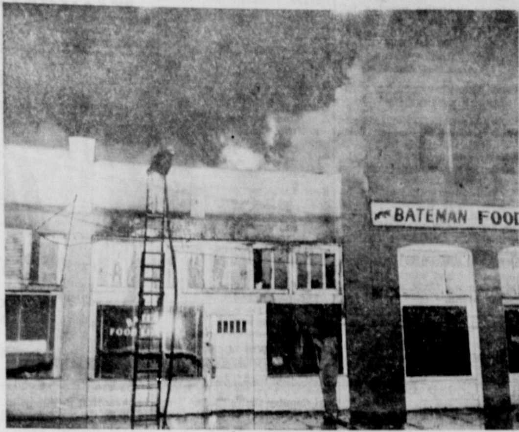
Volunteer firemen are shown attempting to halt flames spreading from Bateman Food Lockers into the City Grocery & Market Wednesday morning. This picture was taken early, and the blaze later gutted the adjoining building. The upper story shown on the right contained the living quarters of C. A. Reed and family. Mr. Reed was owner of the buildings.
