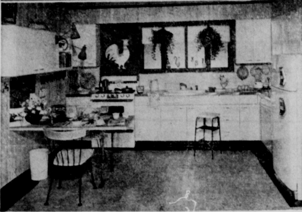
Kitchens with the special Southwestern accent of spaciousness will highlight the Lone Star Gas Company exhibit at the State Fair of Texas in Dallas, October 10-25. This "Chicken Kitchen," with its yellow cabinets, automatic gas range and refrigerator, derives its name from its unusual motif of hens and
