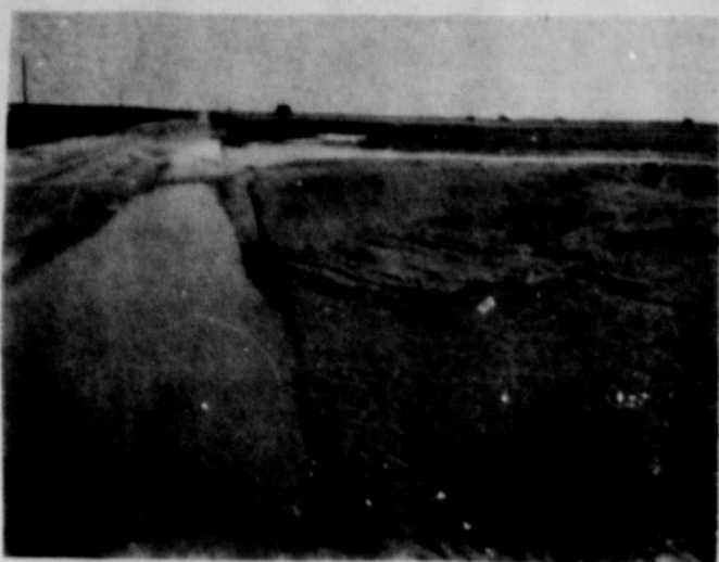
PICTURED HERE: Silt accumulation along a highway following recent heavy rains in this area.
