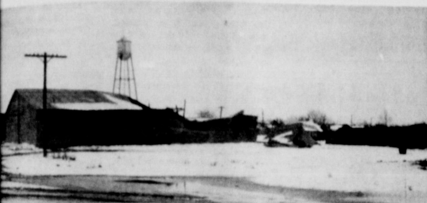
HOUSE where Farmers Grain Co.'s equipment was stored just south of the Brazos River. The building began collapsing Sunday morning after Knox City's BIG snow! There is some damage to any equipment damage, but it is evident by the above photograph that the building was heavily damaged.
