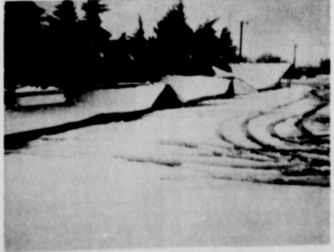
HOSPITAL CARPORT that has sheltered cars of Knox County Hospital employees for several years buckled under the weight of the eight-inch snow Saturday and cars were moved before the structure was flattened.
