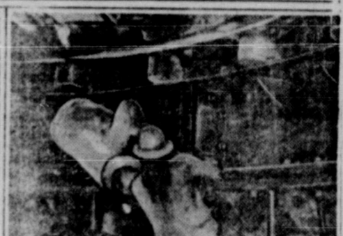
COMPRESSED AIR keeps the river away. Increases in pressure cut down the amount of time men are permitted to work. Two 45-minute shifts a day will be tops when maximum pressures are reached.
