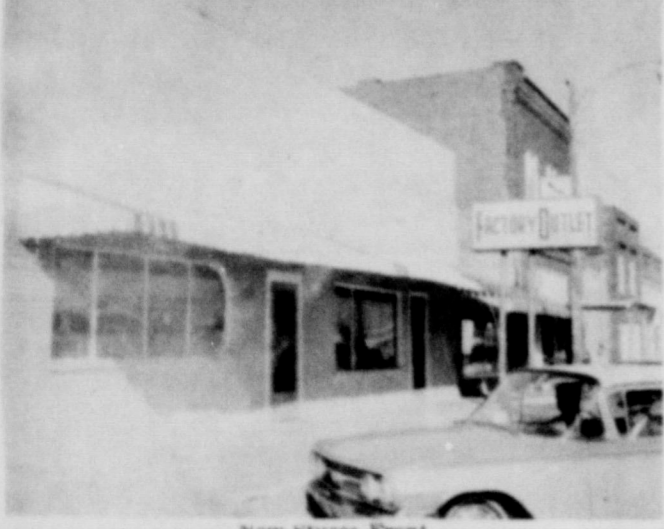
New Stucco Front
