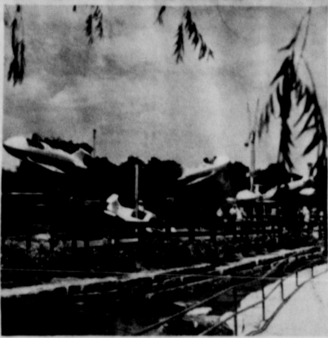
New ride called the Jet Set has just been completed at Six Flags Over Texas. The sophisticated electro-hydraulic steering system enables guests to "fly" these scaled-down models almost exactly like regular aircraft by climbing, banking right or left and diving, responding to the commands of the "pilot" working the control stick.
