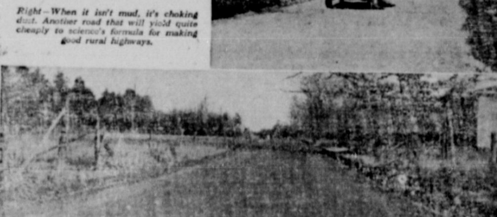
Once not more than a mud road like the one pictured above it, this Virginia thoroughfare resulted from the proper mixtures of local soil materials and calcium chloride to give a "stabilized" surface of the type recommended by the U. S. Bureau of Public Roads for low-cost, all-season purpose.
