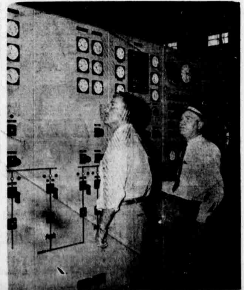
More Power On The Lines—C. O. Holt (left), Plant Chief Engineer and G. G. Hardin of the General Engineering Department, Abilene, check the controls at West Texas Utilities Company's new generating station on Paint Creek as the 33,000 Kilowatt Turbine Generator goes on the line following a test run.
