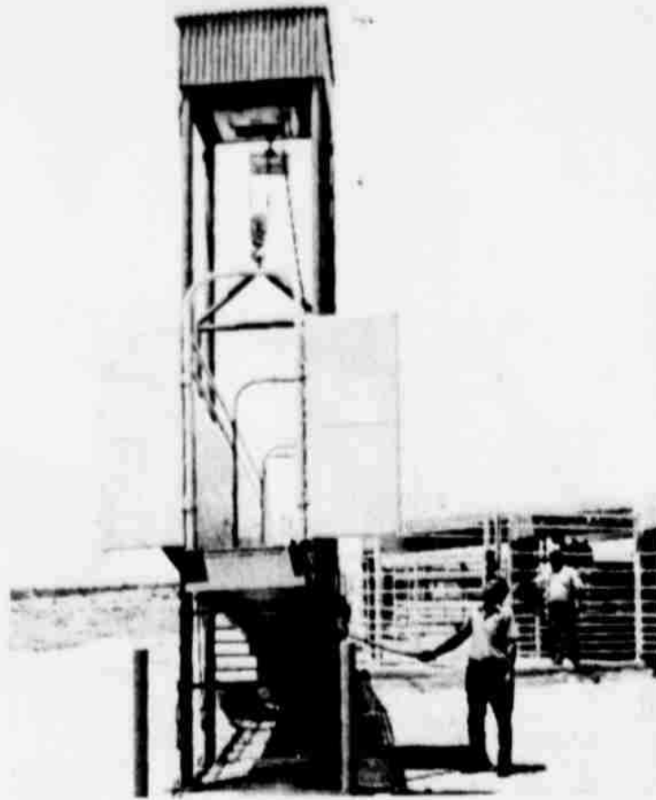
LAREDO EXPORT FACILITIES—Tony Martinez, manager of the Texas Department of Agriculture's newest livestock export facilities in Laredo, demonstrates the operation of a new electrically-operated chute which allows easy movement from one level of a livestock truck to another. The Laredo pens, like the export facilities in five other Texas cities, enable cattle being exported to Mexico to be examined before being shipped across the border.
