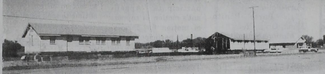
The old barracks building has been set apart, and foundation laid from one end to the other. When complete, the gap between them will be filled to make one solid building 190 feet long with 10 stores that will be "Ol' Town" shown in the drawing.
