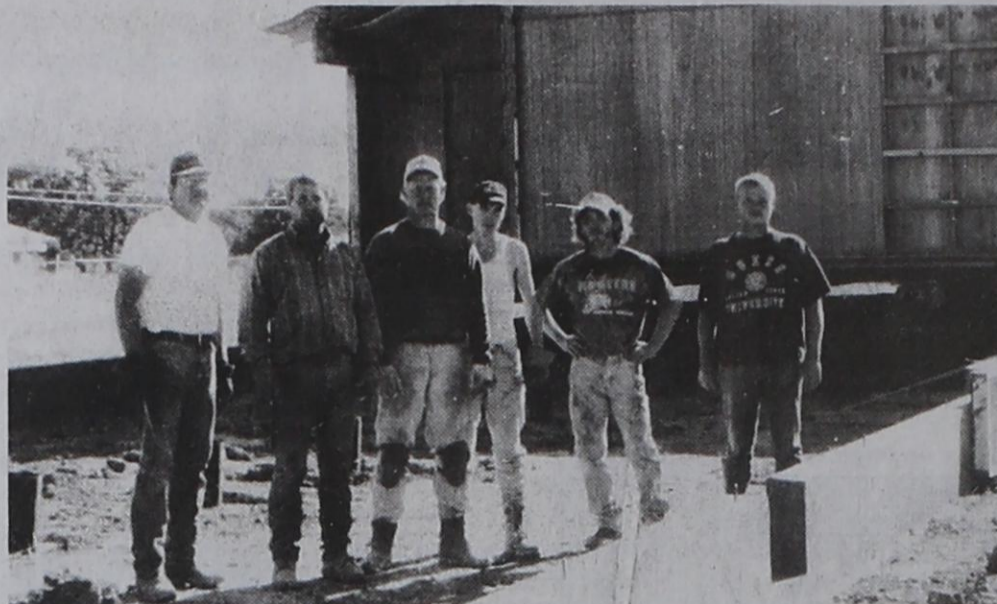
"Ol' Town" Heritage Center Cement/Foundation Workers are Winkle Hawkins, Jimmy Trammell, Dee Sharpe, Will Smeltzer, Fred Andrus and Terry Warner.
