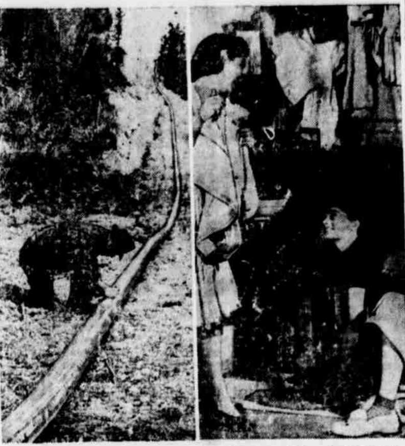
Oil for traffic using the new Alcan highway will be piped 550 miles from the huge underground lake of petroleum resources in the Mackenzie basin at Fort Norman. It will also serve ships along the Alaskan shore. Left: An inspector checks the welding on a section of the line. Right: Two of the many girls working in connection with the project are pictured in their laundry.
