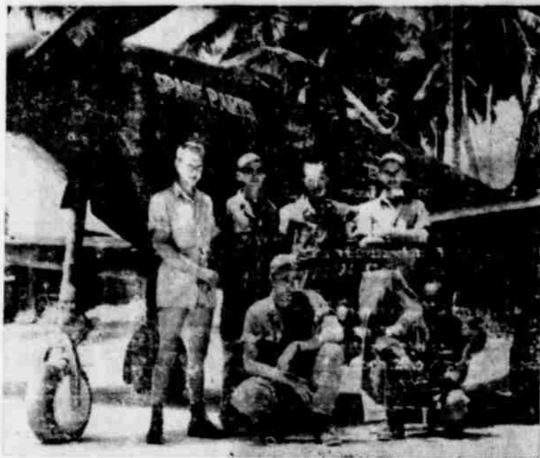
"Spare Parts" is the name of this reborn Bell P-39 Airacobra fighter. Riddled by Jap bullets in the South Pacific, it was tough enough to be patched together again with odds and ends after officers at first thought it was ready for the junk pile. The picture is an official U. S. Air Forces photo and shows some of the men who put their spare parts to good use.
