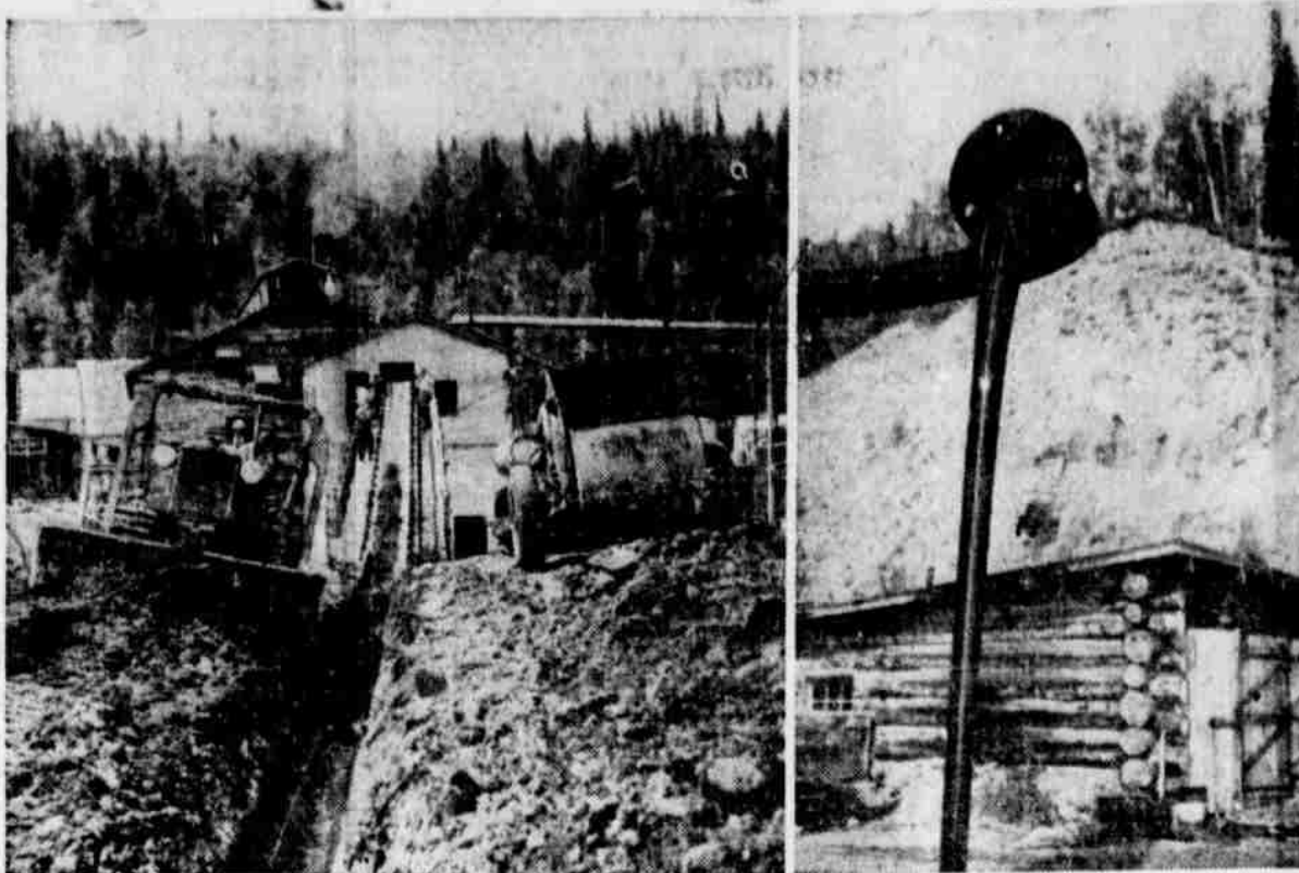
Ten thousand square miles of prehistoric, mineral-rich oil sands in Alberta, Canada, will provide the United Nations with huge quantities of oil. Experimental production has been in effect for more than a year at McMurray, 300 miles northeast of Edmonton. Photos show (left) conveyor belts carrying oil sands to the separation plant where, through flotation, hot water washes oil free from sand. Right: "Black gold" flows freely through the pipeline after the separation process is completed.
