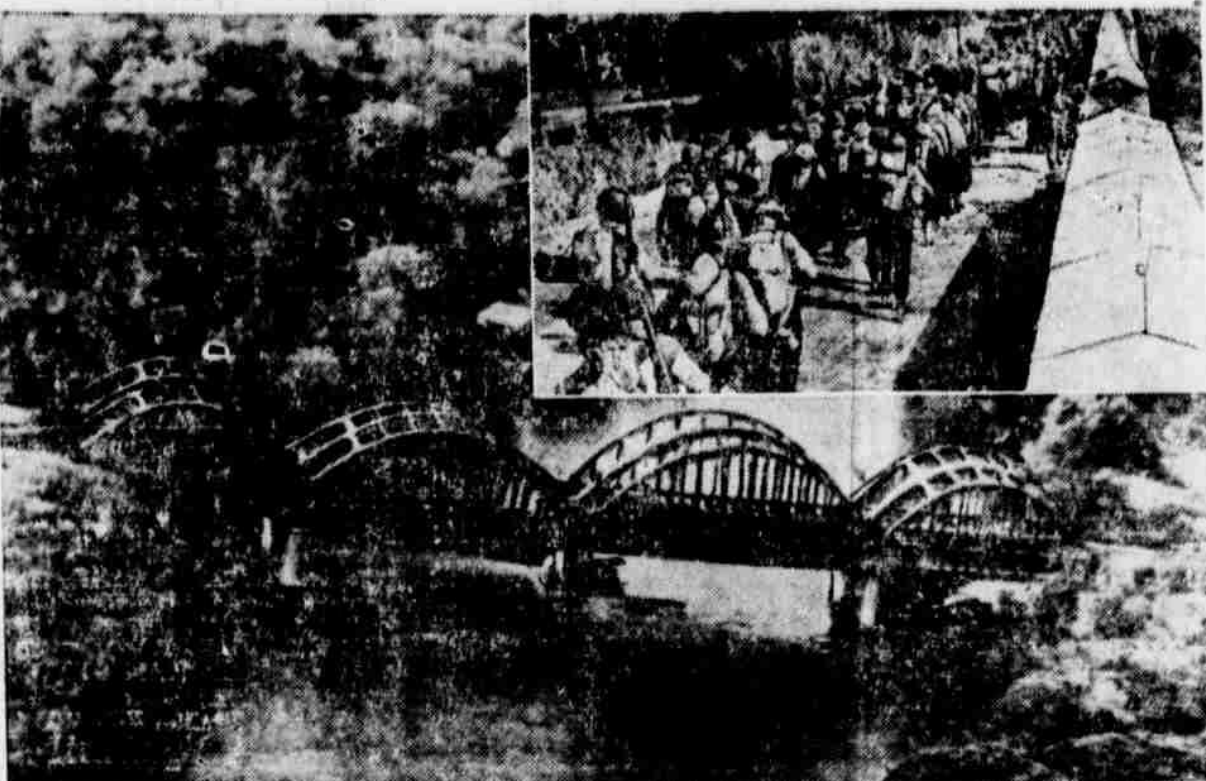
This railroad bridge, east of Toulon, was demolished by the retreating Huns as Allied forces continued to push steadily inland on the southern coast of France. The Nazis left little in the way of railroad tracks or bridges or highway for the advancing Allied armies...
