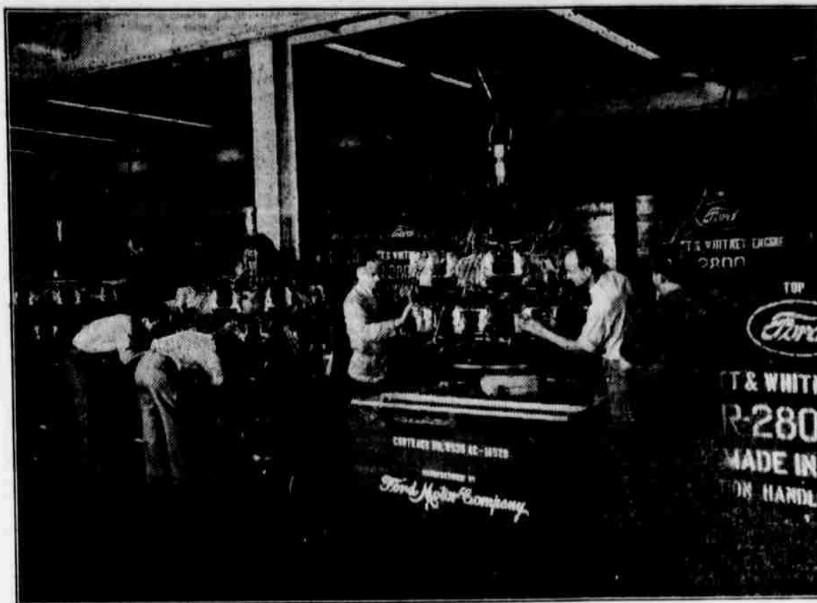
DEARBORN, Mich.—This is a corner of months in this new aircraft unit of the Ford Rouge plant. Another major Ford defense project is the contract to build big four-engine Consolidated B-24 bombers. A $58,000,000 plant is under construction for this job at Willow Run, near Ypsilanti, Mich.
