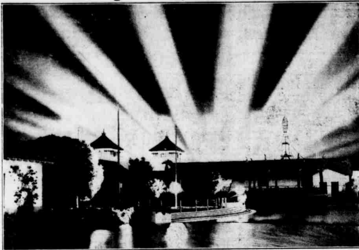
These penetrating fingers of light point across Treasure Island skies each night of the 1940 Golden Gate International Exposition. Silhouetted in the foreground is the Japanese Pavilion bordering the mirrored lake, which is the Lagoon of All Nations at the Fair.
