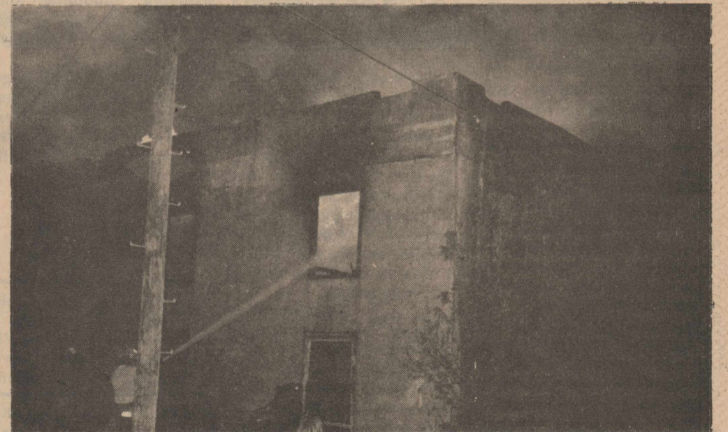
THIS OLD BUILDING in downtown Knox City was completely ablaze in the upstairs southeast corner when firemen arrived on the scene at 7:00 p.m. Sunday, but with the help of neighboring Benjamin and Munday firemen, the blaze was contained to about six rooms by 10:00 p.m. Firemen remained on the scene until midnight to make sure the blaze did not break out again in the business district.
