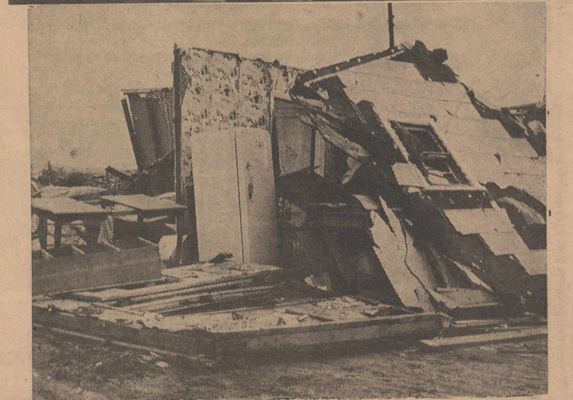
THESE TWO PICTURES were taken May 24 after Olton had been struck by a devastating tornado. One shows Mr. and Mrs. R. A. Ragle at the rubble-strewn site of their home. The other is a house in south Olton. It was lifted off its foundation and left sitting in the street in front of Bohner Baptist Church.
