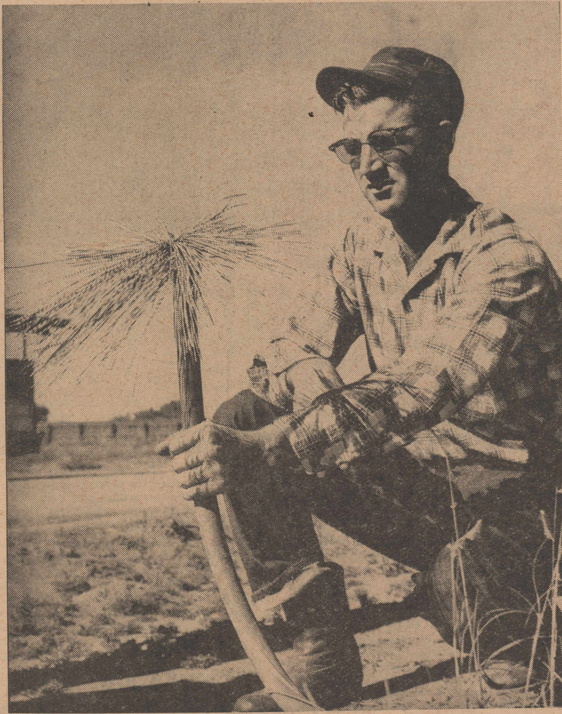
Denver Offield, General Telephone service man in Olton, holds a cable containing 606 telephone wires which must be spliced. The cable was snapped by an A-frame truck operated by Duward Price. Telephone service was out to Hillcrest Addition for about one day. The accident occurred Monday shortly before noon. The entire cable section had to be cut out and a new section replaced. That makes 1,212 wires to be correctly joined. (STAFF PHOTO)
