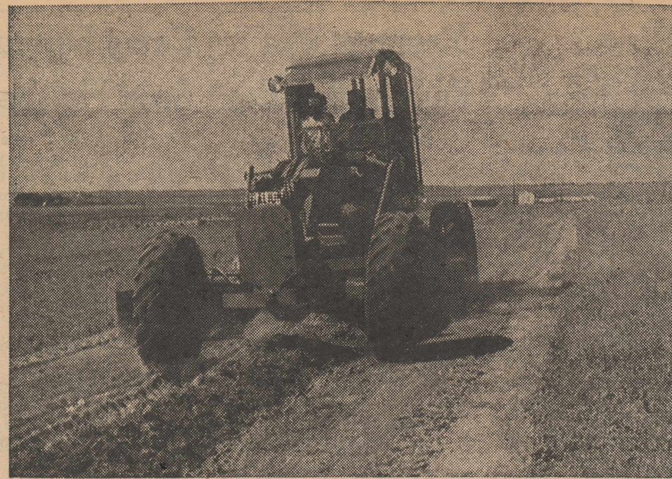
WORK was going forward on the Olton Municipal Recreation Center this week. A maintainer is shown here grading out a road across the 90-acre tract being improved into a playground. (STAFF PHOTO)
