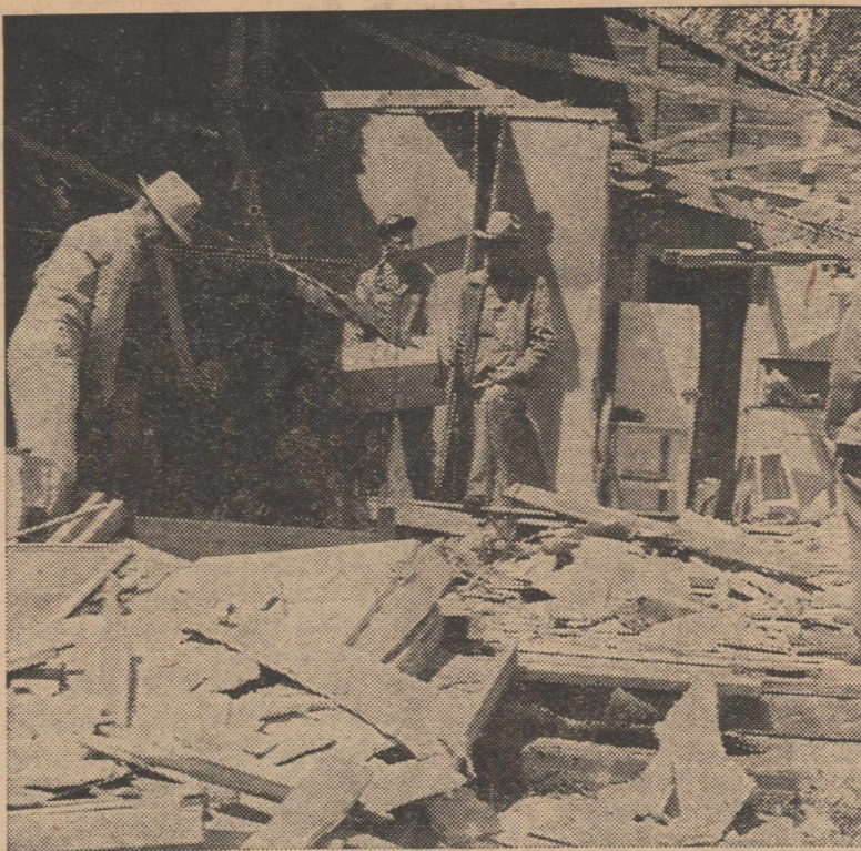
NEIGHBORS PITCHED IN to help the S. O. Owens' salvage as much as possible from their tornado-struck home. Here an unidentified gentleman manhandles a set of bed springs. (Enterprise Photo)
