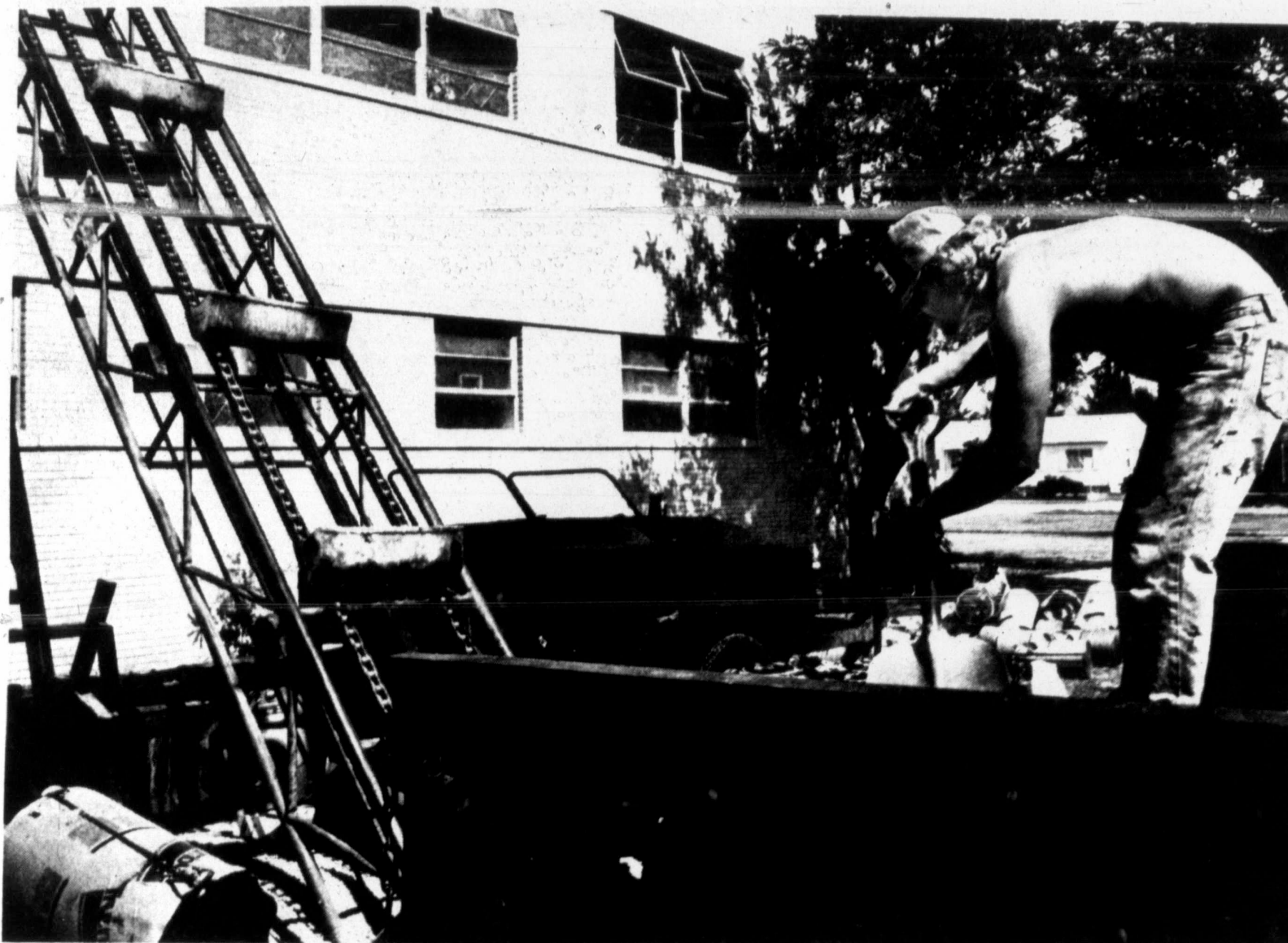
GRAVEL — Keeping up with a gravel-lifter was hot work for Jeff Bogle of Texas Roofing Co. of Lubbock last week outside the Snyder High School auditorium, where workmen were re-tarring a roof. (SDN Staff Photo)
