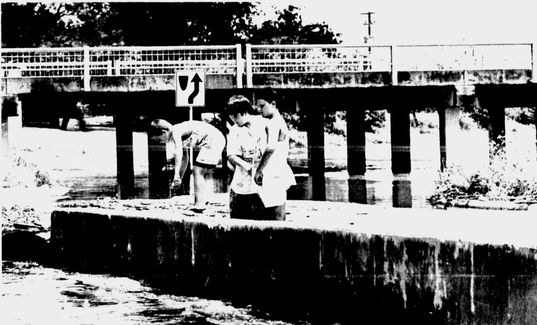
WATER, WATER EVERYWHERE — Deep Creek was still gushing early Monday afternoon at the 28th St. bridge, having swamped the street under the overpass, after a night and morning of rainfall. In-
