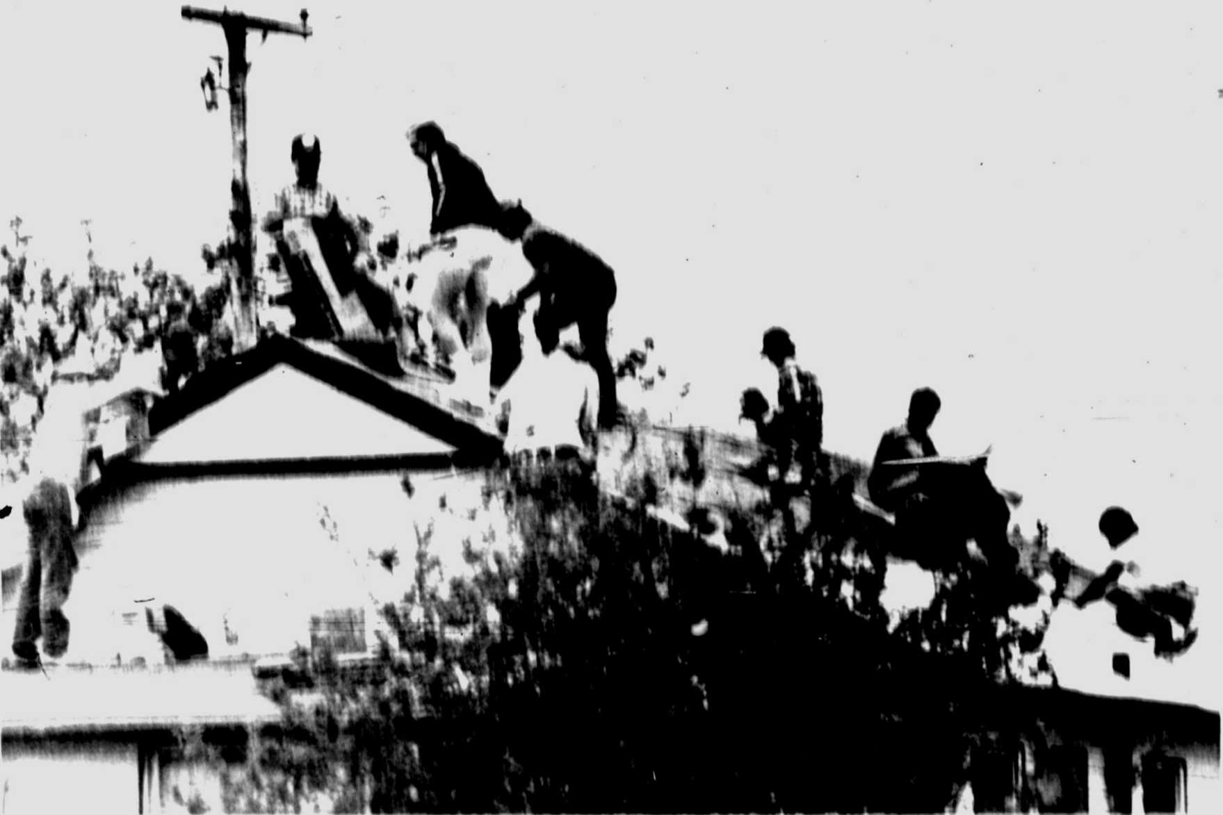
A NEW ROUTE — Chevrolet USA employees here among an estimated 100 volunteers working here Saturday to renovate the homes of elderly and disabled persons. This group is shown re-roofing a house, one of seven repair projects undertaken during the day. The effort
