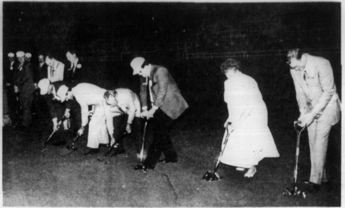
GROUND-BREAKING — Leaders of local financial institutions were among those who broke symbolic ground with silver-plated shovels Monday at Scurry County Coliseum for the new Texas Department of Corrections unit. They were, from
