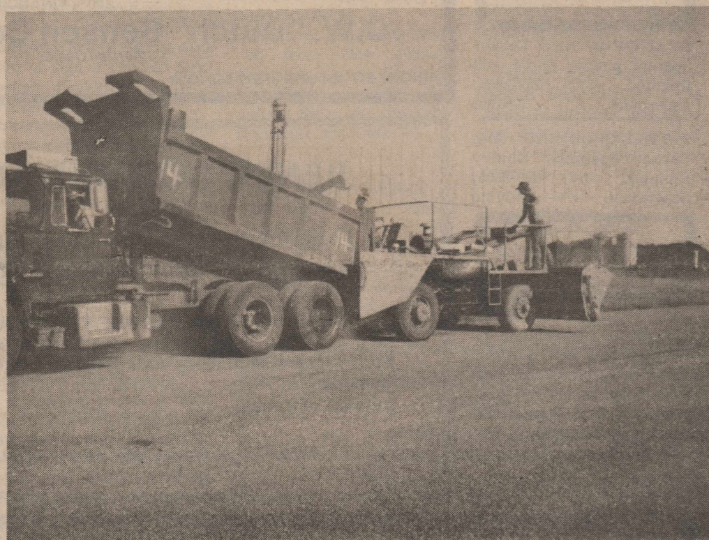
SEALCOATING OF The Landing Strip at Knox City Municipal Airport began last week as part of the airport grant. West Texas Construction Co. of Abilene crew began the hot topping Thursday. According to city officials, wiring on all the lights will be done within the next six weeks to complete the airport project.
