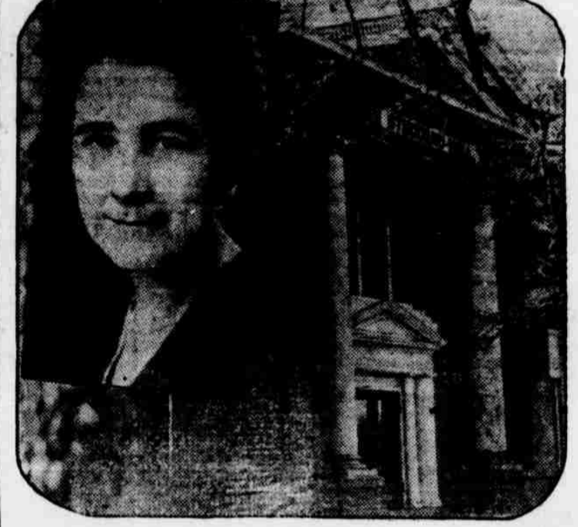
President L. H. Hubbard, pick in hand, begins wrecking of Stoddard Hall, first state dormitory at Texas State College for Women (TSCW), which will be replaced through PWA grants by a modern four-story, fireproof building. The lower picture shows old Stoddard in all the glory of former days, and (inset) Miss Jessie H. Humphries, its first director, now associate dean of the college.
