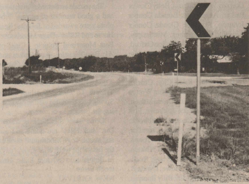
NEW CHEVRONS have been placed at the curve on State Highway 222 west of Knox City.
