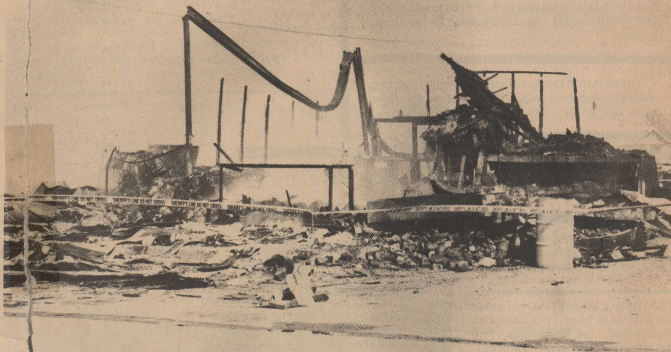
ALL THAT REMAINS of Dub's Grocery and Station in Benjamin is this pile of twisted metal and ashes after a fire completely destroyed the business early Sunday morning. Still smoking when this photograph was taken late Sunday afternoon, the grocery store and bus station was the longest continuously run business in the community of Benjamin. Owner Dub Cartwright indicated that he would not rebuild the business. (News Photo)
