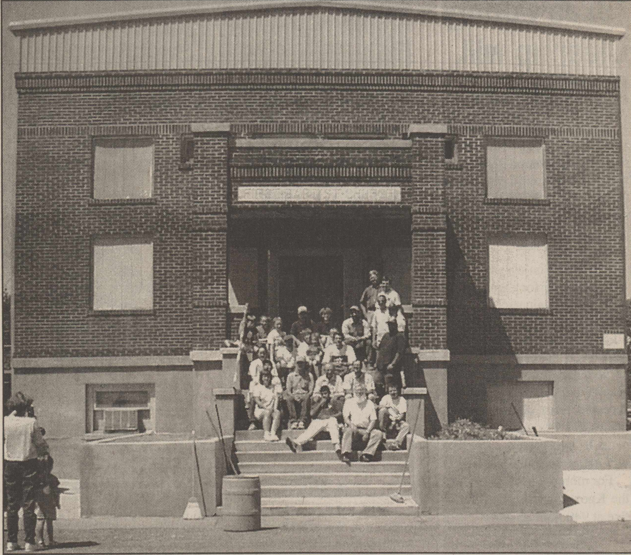
A LABOR OF LOVE was carried out at First Baptist Church, Knox City, this past weekend as members of CIA (Christians In Action) mission group unselfishly worked to restore the second floor roof of the newly named Family Life Center at the corner of South Second and Central. Workers were housed with various church members and were from pastor Johnny Johnson's hometown of Perryton. The workers now live in various parts of the South Plains, Texas Panhandle and Oklahoma but were once residents of Perryton. The group began their project on Thursday evening and continued through Saturday afternoon. They shared and worshipped with the congregation on Sunday morning and were honored with a covered dish luncheon Sunday noon before their departure. (NEWS digital photo)
