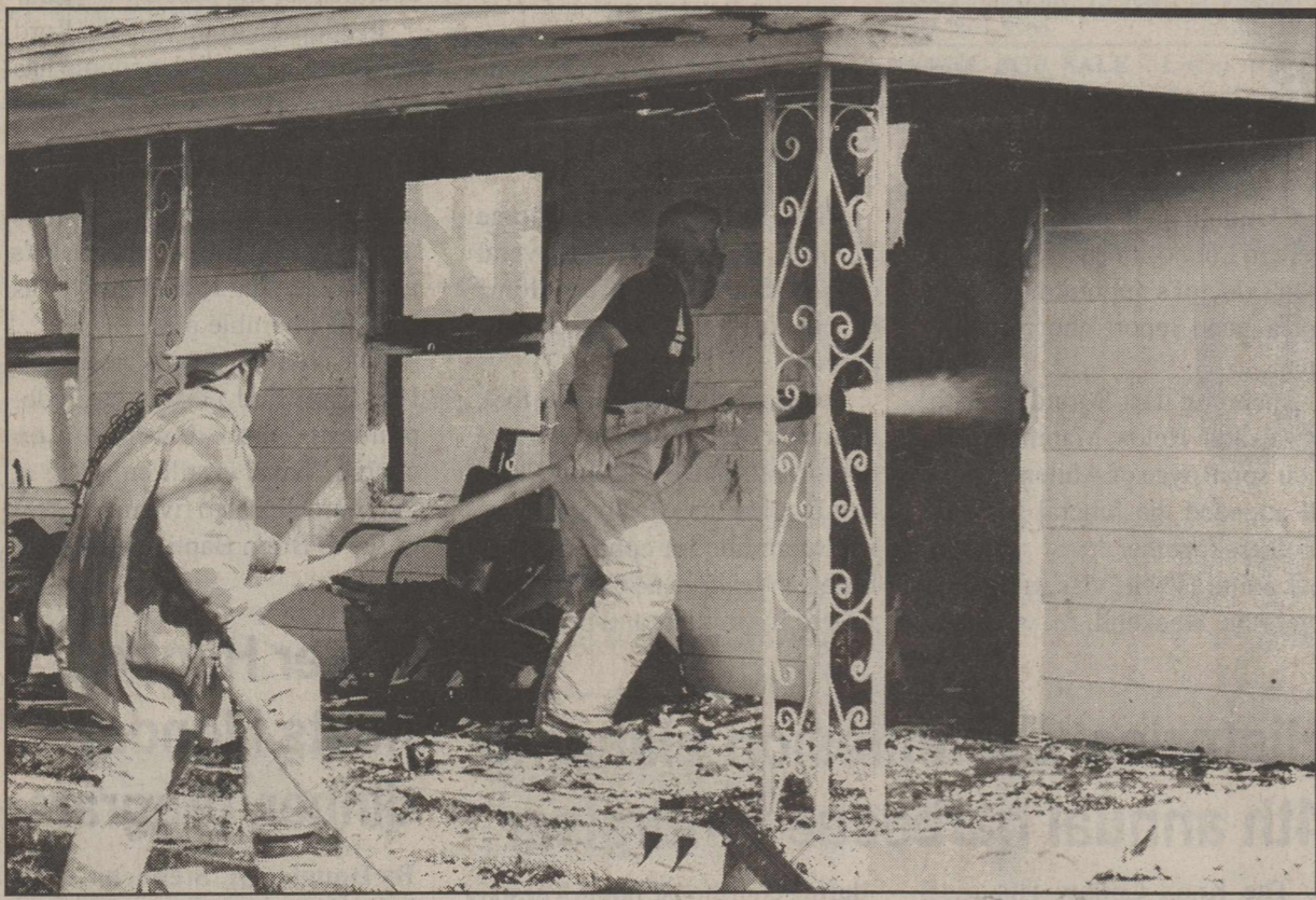
BATTLING THE TRAGIC FIRE last Saturday at the residence of Jack and Romain Stubbs, Knox City Volunteer Firemen (left to right) Douglas Stephens and Harry Steen are shown here as they direct water in to the front door area on the west side of the house. Despite the efforts of volunteer firemen from Knox City, Rochester, Munday and Benjamin, the residence was considered a total loss.
