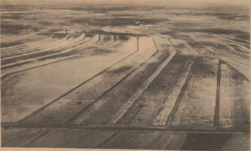
73610 Ft. Of Paraller Terraces Were Constructed
