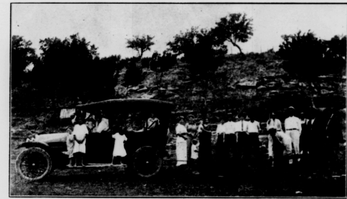
BREAKING DIRT FOR THE NEW M. E. CHURCH, SOUTH.
